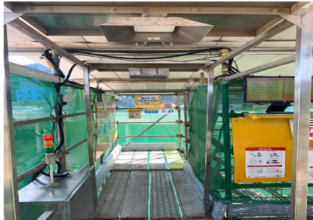
Overview of a RFID gantry with a live tally board visual display. Electronic records aids contact tracing
