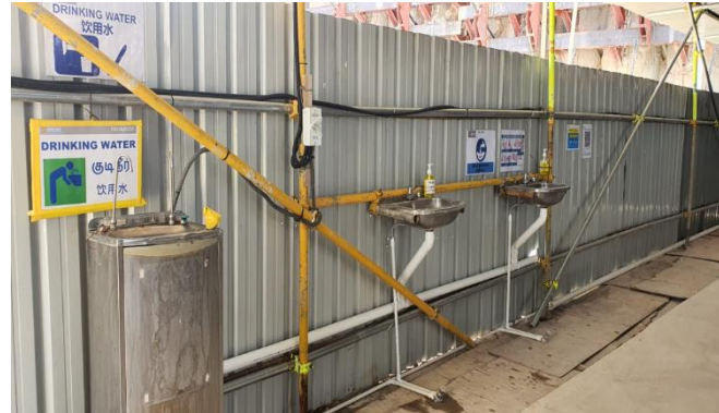
On site rest area with hand wash facilities beside drinking water point
