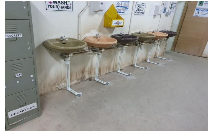
Handwash area with foot paddle at the canteen toilet
