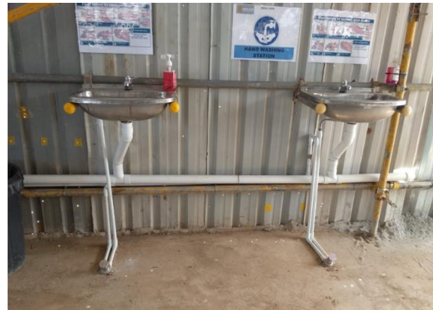
Handwash area with foot paddle at site rest area
