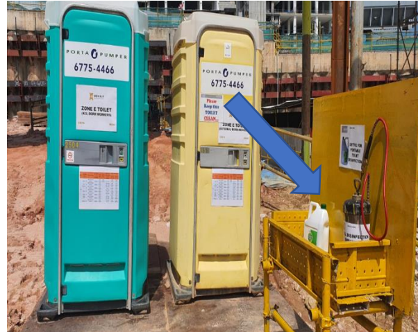
Disinfectant provided for all site toilets
