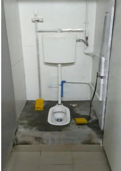
Toilet flushing (stepping on the yellow plate) without worker to press the flushing button
