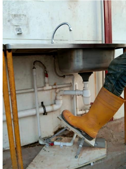
Washing point (stepping on the plate underneath) without worker to turn off / on the tap
