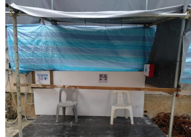
Sick bay not fully enclosed or not provided
