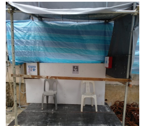
Poor isolation facility for sick workers 患病工人的隔离设施差
