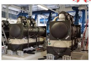
**Magnetic bearing centrifugal chillers** Rotating shaft levitating on a magnetic field eliminate mechanical friction loss and allow lubricant-free operation. Reduces maintenance costs and provides energy savings of up to 57%.
