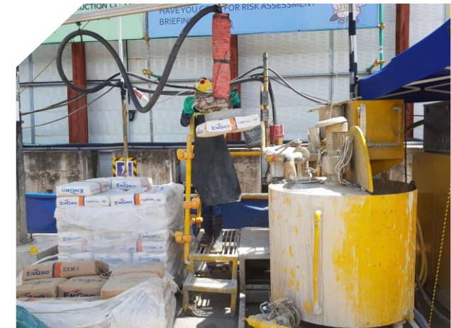
Mechanical Lifting of Cement Bags
