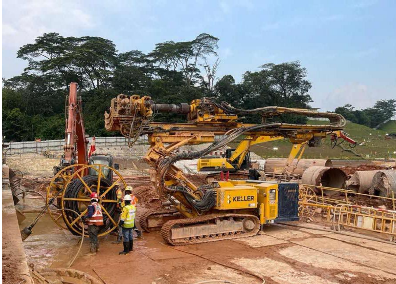
360° Rotation Mechanical Handler to Carry and Install Ground Anchors
