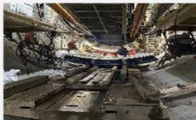
(c) Automatic Placement of Segment in the designated location at the Segment Feeder
