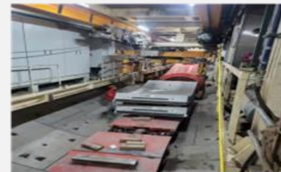
(a) Automatic Hoisting of Segment once it is in position from Quick Unloader
