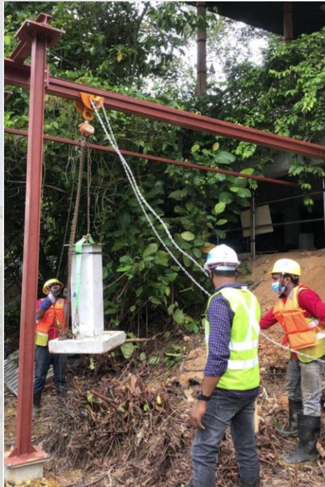
Gantry & Chain Block (Pulley System) only used at localized terrain
