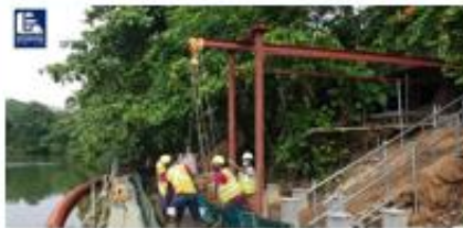
Unloading of footings on a slope area
