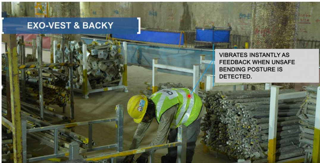
BACKY Vibrates when worker has improper posture
