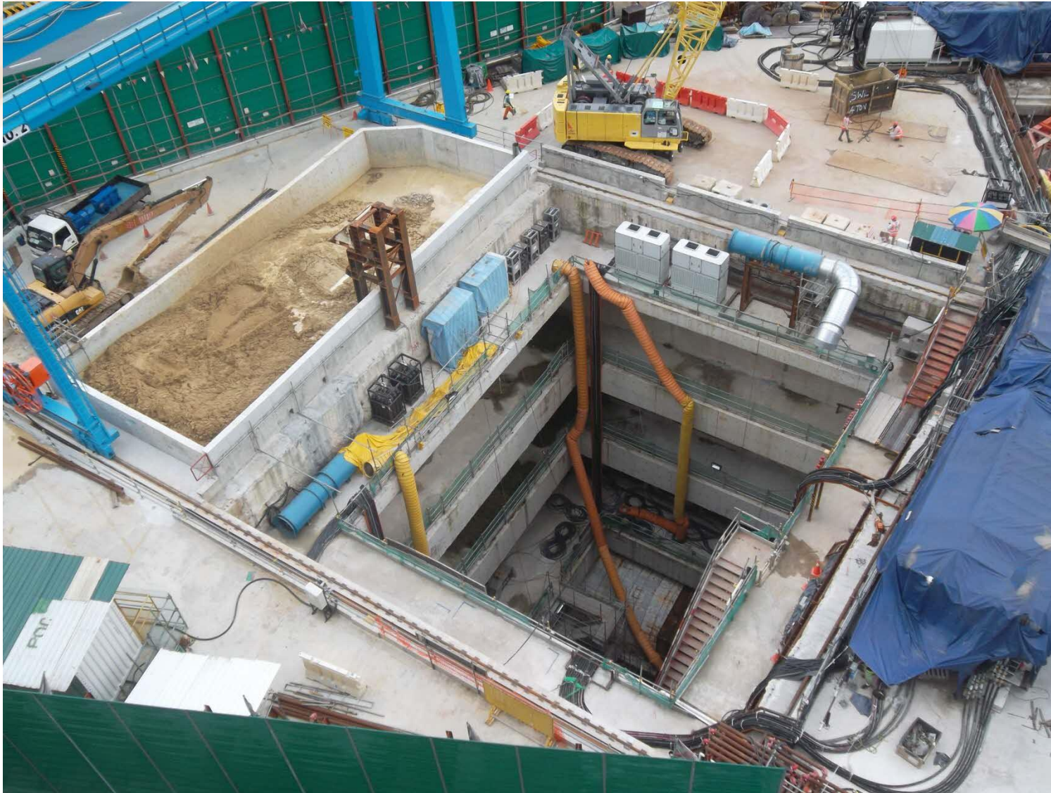
Space limitations to handle 2 TBM in the shaft
