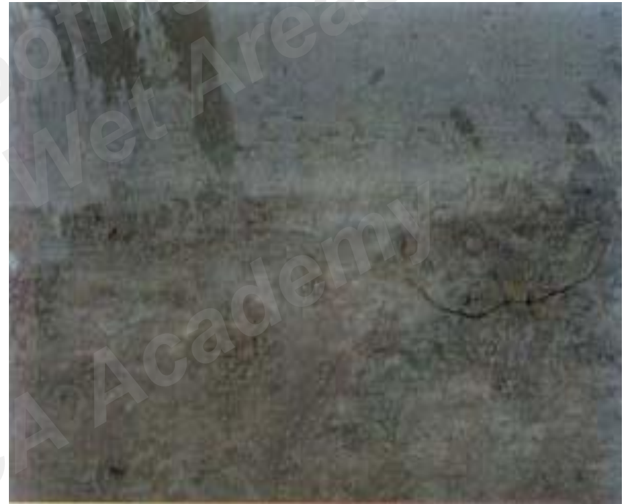
Figure 2.4.1: Examples of foreign materials on concrete surface Efflorescence Surface Laitance
