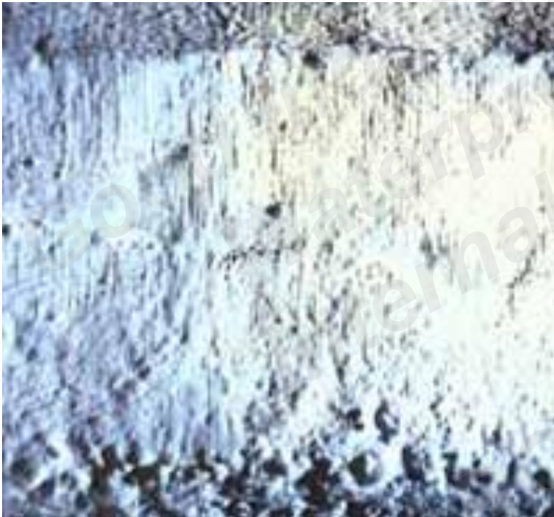
Figure 2.4.1: Examples of foreign materials on concrete surface Efflorescence Surface Laitance
