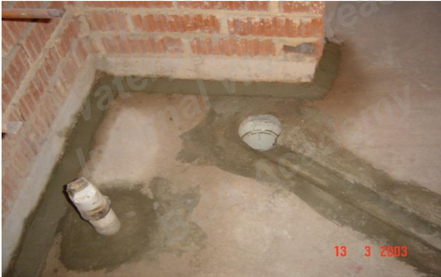
Fillet around pipe penetration
