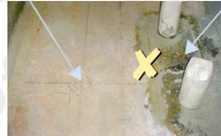
Tile marking for pipe location
