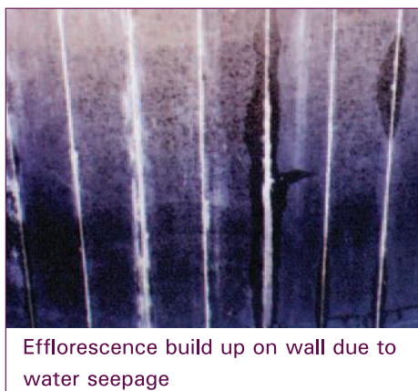
Leakage on the ceiling and walls below and adjacent to wet areas
