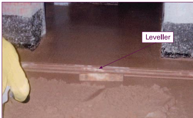
Figure 7.6: Screeding in progress
