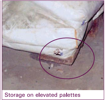
Figure 4.1: Storage of waterproofing products on site
