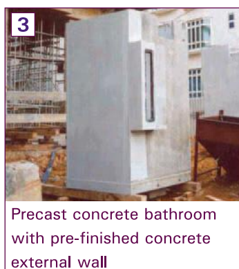
1 Pre-assembled bathroom cell prior to delivery
