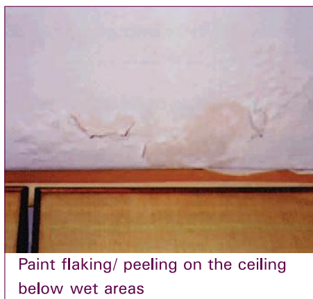
Leakage on the ceiling and walls below and adjacent to wet areas
