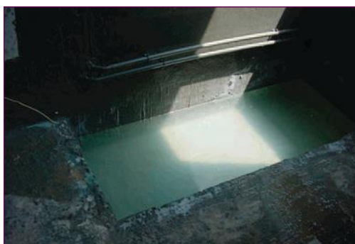
Watertightness test at sunken bath
