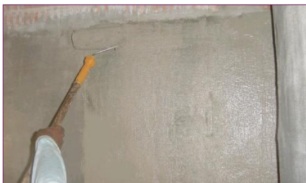
Roller application to wall
