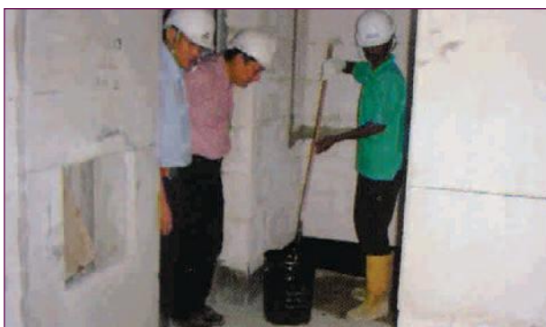
Joint inspection during application
