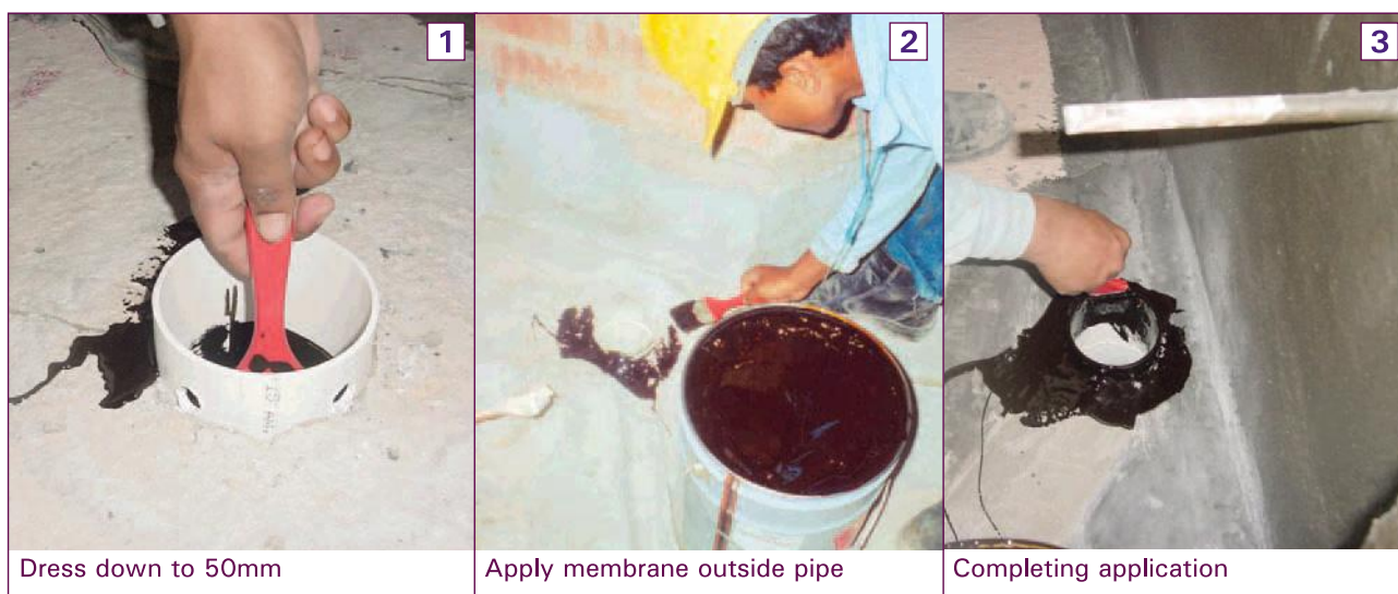
Figure 6.8: Application of membrane at floor outlet
