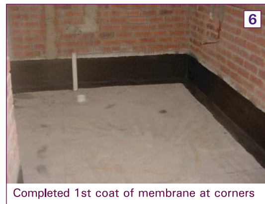
Figure 6.6: Application of waterproofing membrane around wall-floor junctions
