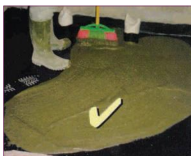
Figure 6.3: Apply using broom
