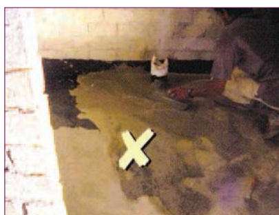
Figure 6.2: Apply using steel trowel
