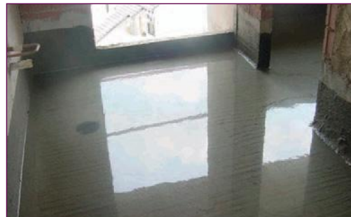
Watertightness test after membrane application
