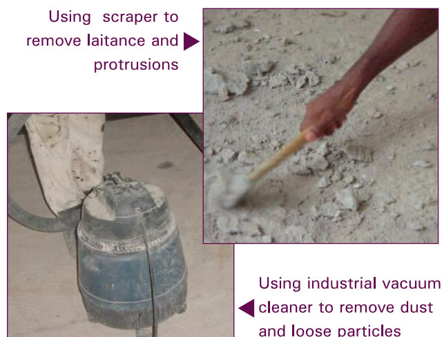
Figure 5.3: Examples of concrete surface cleaning methods
