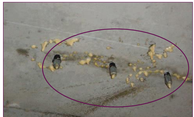
h) Fully grouted crack line
