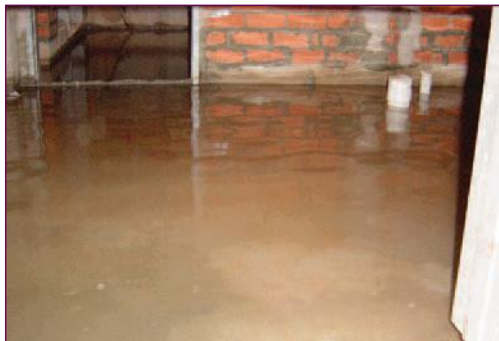
Structure watertightness test
