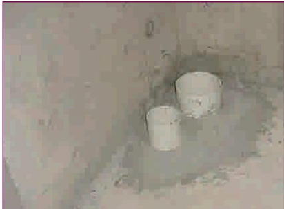
Figure 5.6: Fillet installed around pipe penetrations
