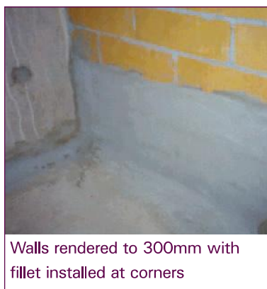
Figure 5.4: Surface preparation to brickwalls and internal corners
