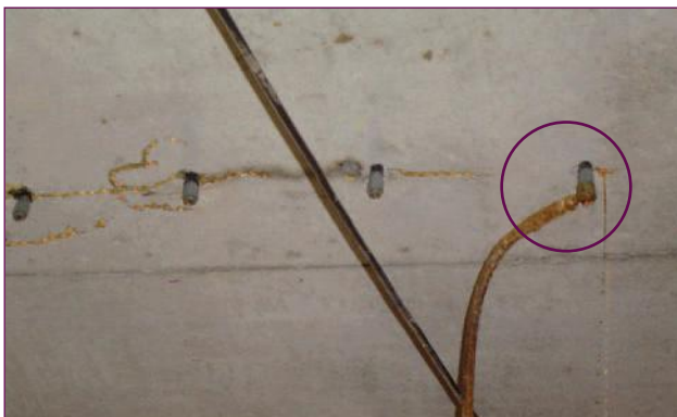
g) Grouting in progress
