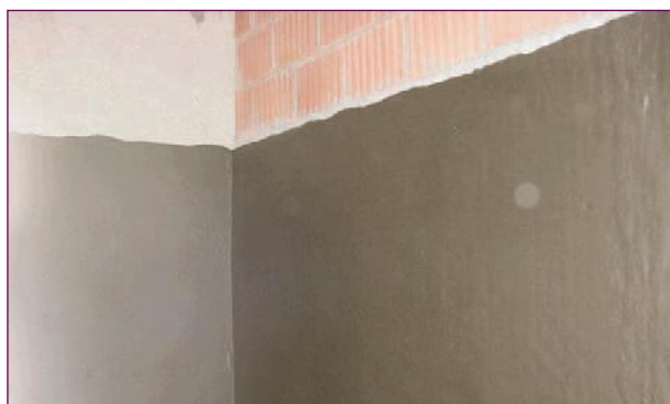
Completed wall application
