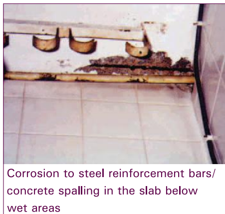
Figure 8.2: Common defects arising from leaks
