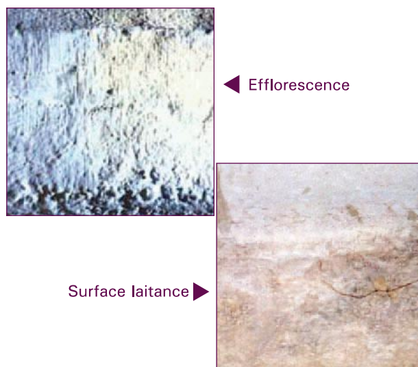
Figure 5.1: Examples of foreign materials on concrete surface
