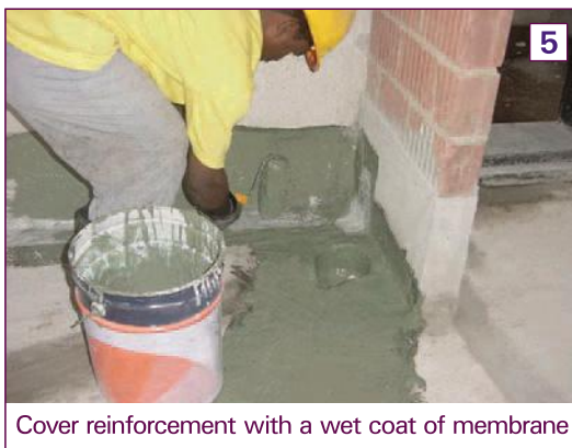
Figure 6.6: Application of waterproofing membrane around wall-floor junctions
