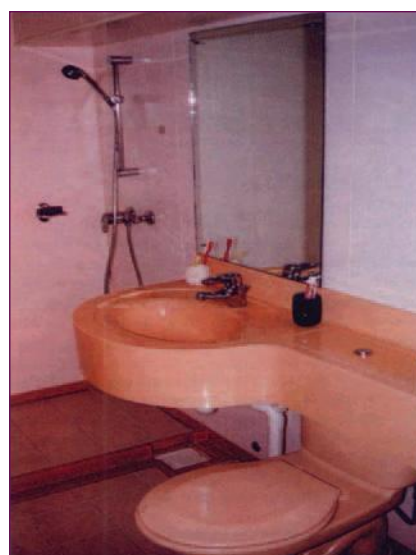
Figure 2.1: Interior of a prefabricated bathroom
