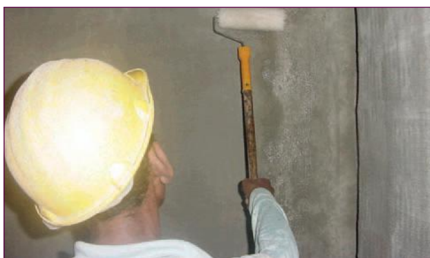
Dampen wall surface with wet roller
