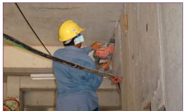
d) Drilling hole
