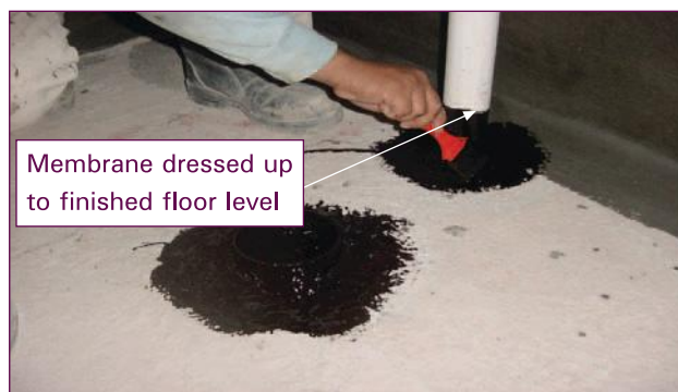
Figure 6.7: Application of membrane at pipe penetrations
