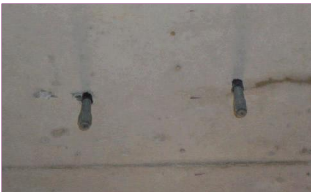
e) Nozzles inserted along crack line
