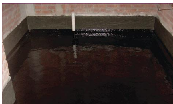
Completed floor application
