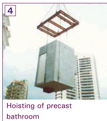
Figure 2.3: Pre-assembled PBUs
