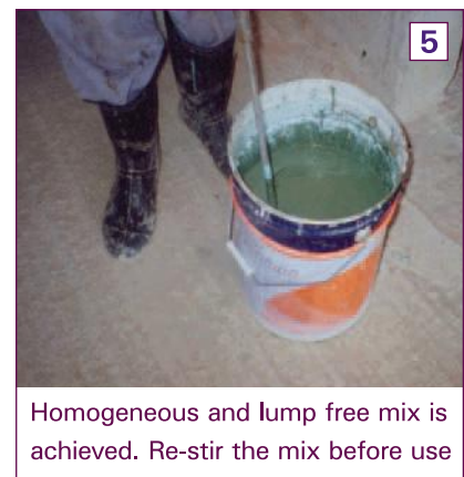
Figure 6.4: Mixing of 2-component waterproofing products
