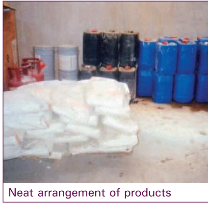
Figure 4.1: Storage of waterproofing products on site
