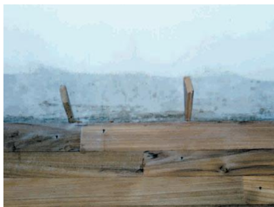
Expansion gap at the perimeter of room
