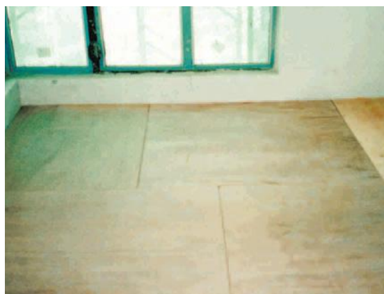
Layout of plywood sub-base in a staggered manner
