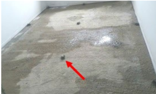
Provide level-pegs before screeding
