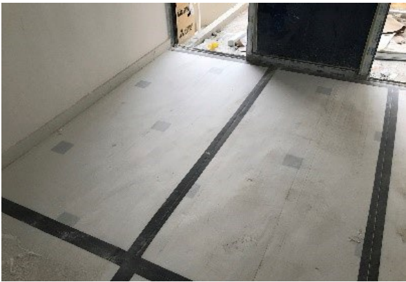
Completed stonework protected with protective material
