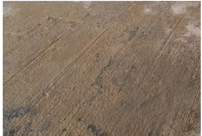
Cleaning surface with water
