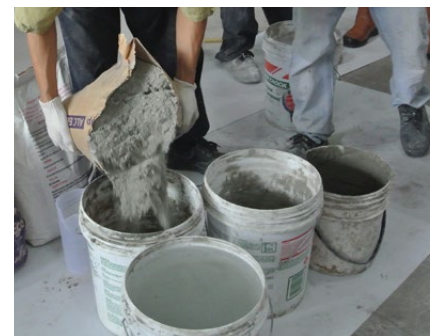
Adding powdered polymer into container
