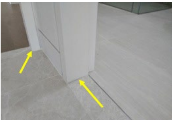
Joint at door frame covered with sealant
