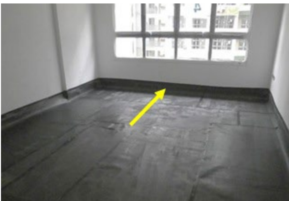
Protection with an up-turn
