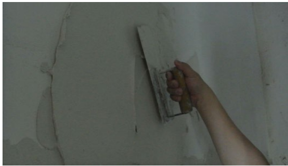
Spreading adhesive with flat side of trowel
