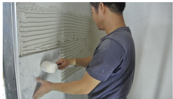
Tapping on stone for uniformity
