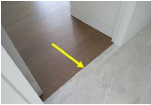
Joint with metallic strip
