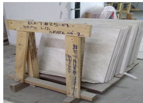
Stones stacked after dry lay
