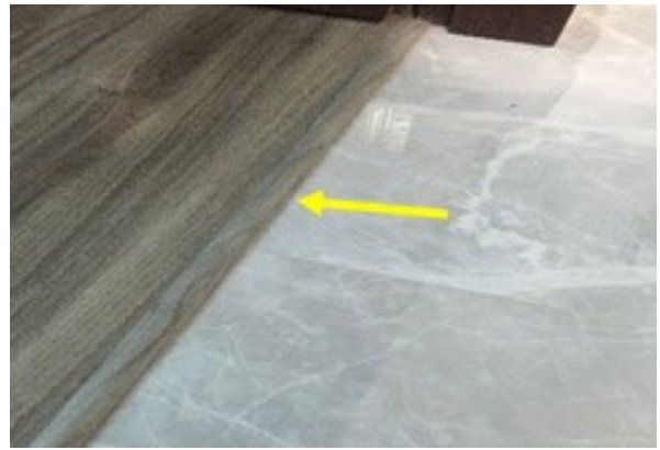
Joint with laminate or timber capping
