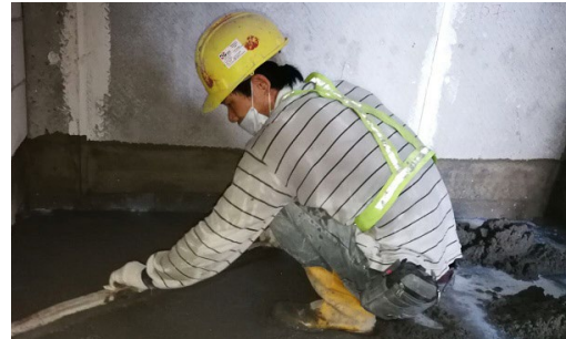
Screeding with timber float
