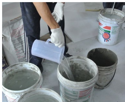
Pouring measured water into clean container
