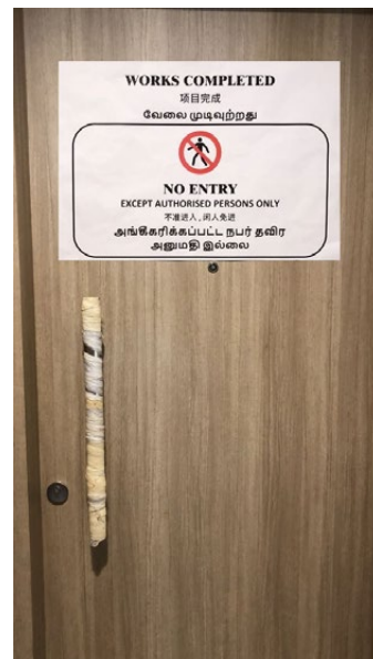
Completed works protected by restricting access
