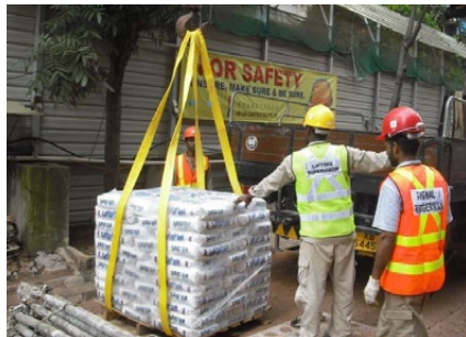
Offloading materials from truck
