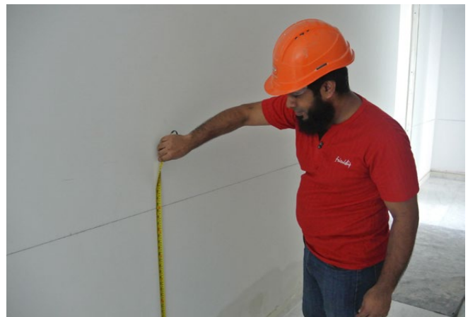
Checking level of surface
