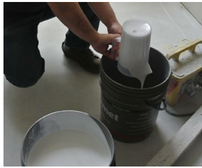
Pouring component 1 into a clean container
