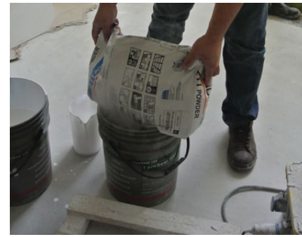
Adding powdered polymer (component 2) into the container
