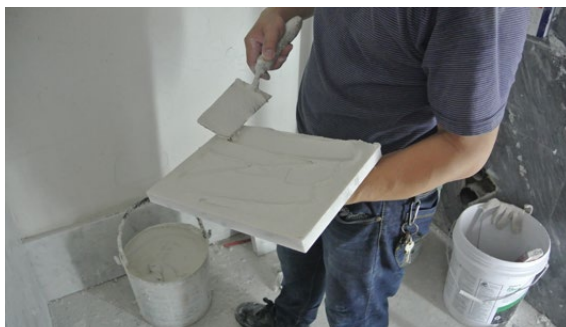
Applying adhesive on back surface of stone
