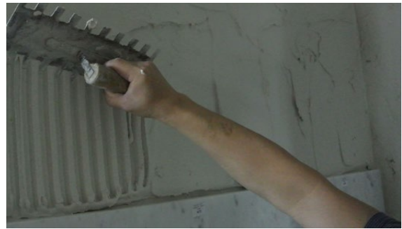
Trowelling adhesive with notched-trowel
