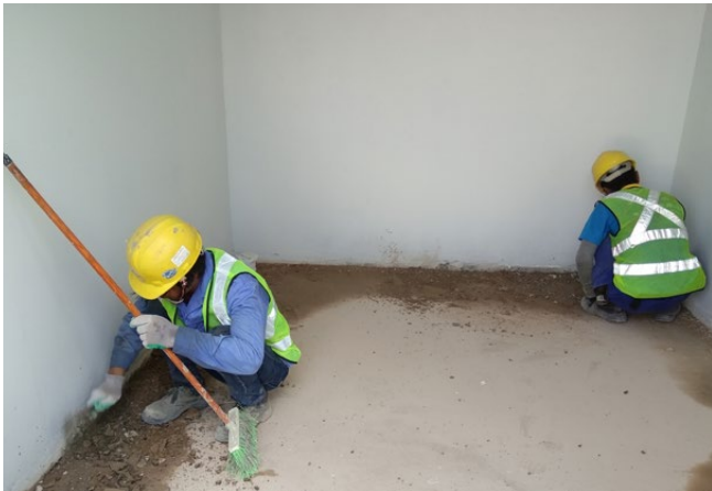
Removing concrete protrusion
