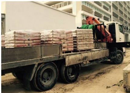
Transporting materials to site
