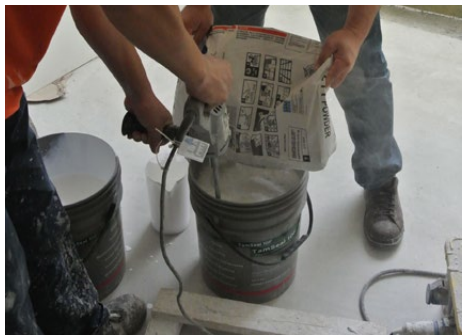
Mixing with electric mixer at low speed
