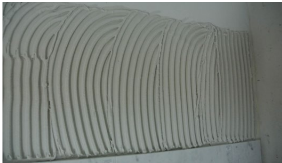
Adhesive fully trowelled
