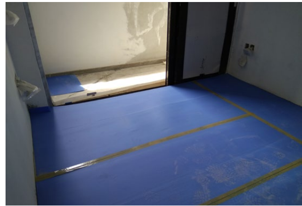
Completed stonework protected with protective material
