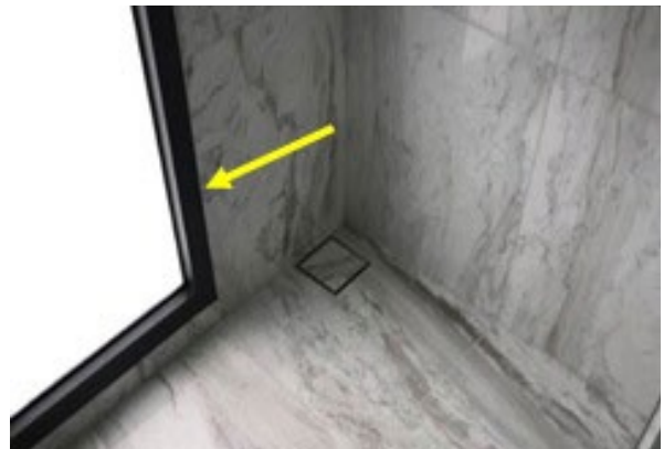
Window frame flush with wall finish surface
