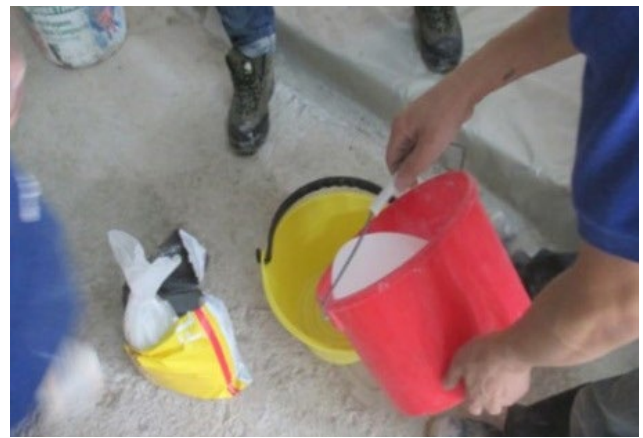
Grout preparation similar to adhesive preparation
