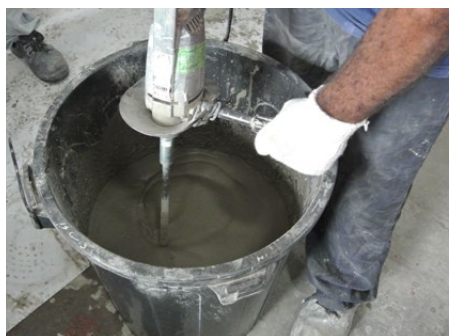
Mixing with an electric mixer
