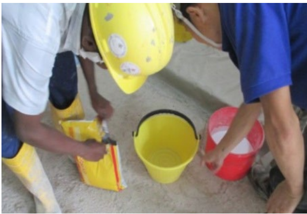
Grout preparation similar to adhesive preparation
