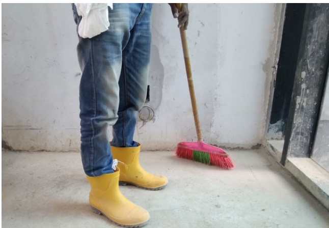
Cleaning surface with broom
