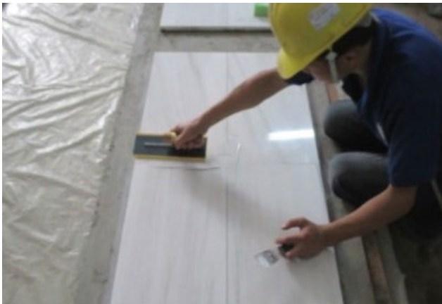
Filling grout joints with firm rubber trowel
