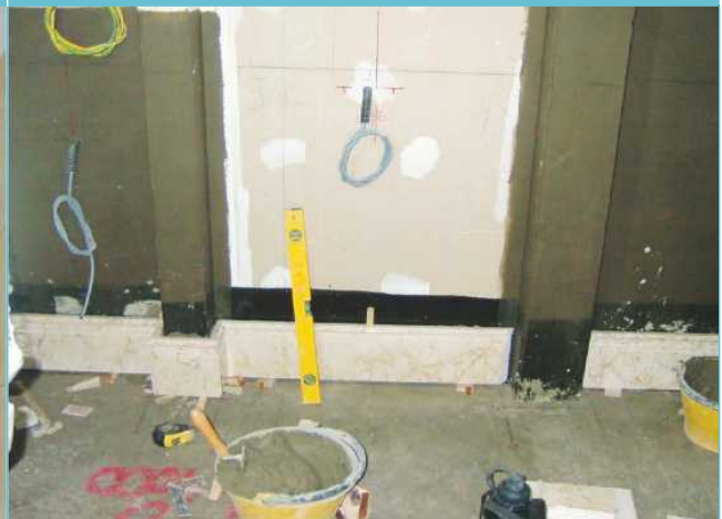
Figure 8.1b Drywall Partition with Waterproofing Membrane
