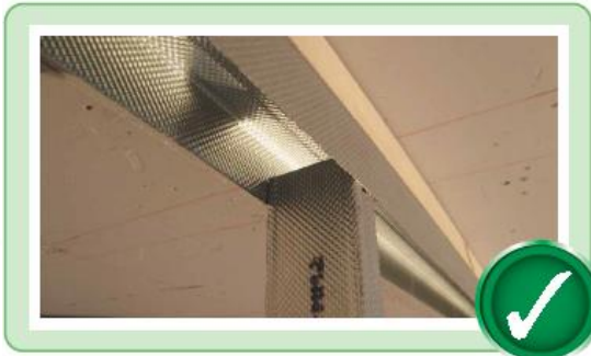
• 25mm downward deflection only, minimum 20mm engagement – stud out short to allow deflection
