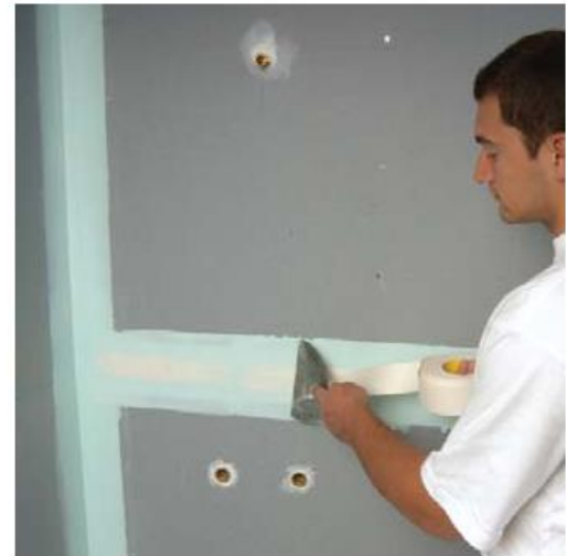
3. Bed in paper jointing tape at sheet joints.
