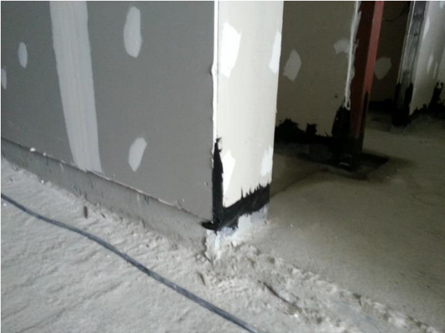
Drywall will fix on the concrete kerb with water proofing..
