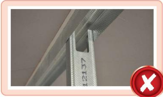
• Service cut-outs should not coincide with head or base channel
