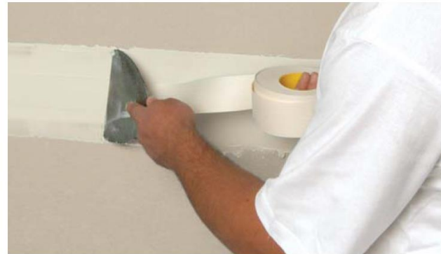
2. First coat - Bed tape
