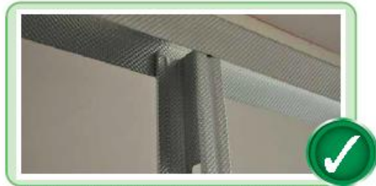
• When deflection heads are installed, do not fix the Cyprane stud into the head track as this will prevent deflection occurring
