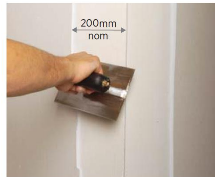
3. Apply second coat to corner faces
