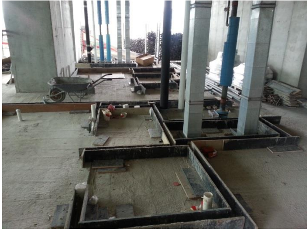
Setting out Kerb at toilet area.
