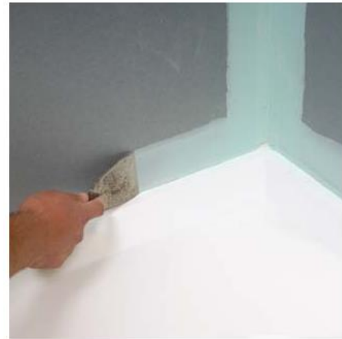
6. Apply skim coat of Wet Area Taping Cement at sheet base.
