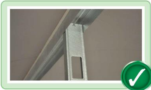
• Cut through solid section of stud profile
