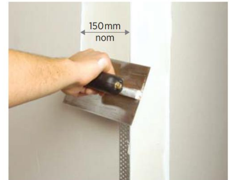
2. Apply first coat to both corner faces
