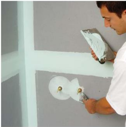
4. Apply skim coat of Wet Area Taping Cement at joints and around penetrations.
