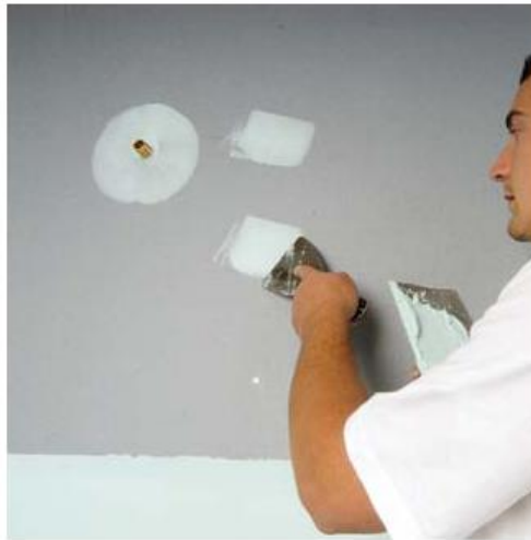
5. Apply skim coat of Wet Area Taping Cement to fastener heads.
