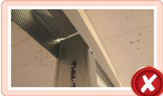
• 25mm downward deflection only – stud too long and will not allow deflection to occur
