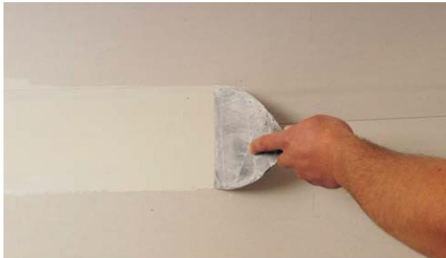
1. First coat - Bedding compound
