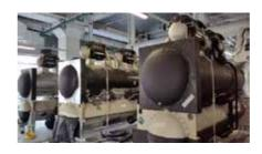
The chiller plant at the Academic Tower roof deck serves two purposes - functional and educational. It is designed as a spacious room so that students can learn about how an efficient chiller plant is designed. This is unlike conventional chiller plants which are congested, dimly lit and where pipes are not labelled.
