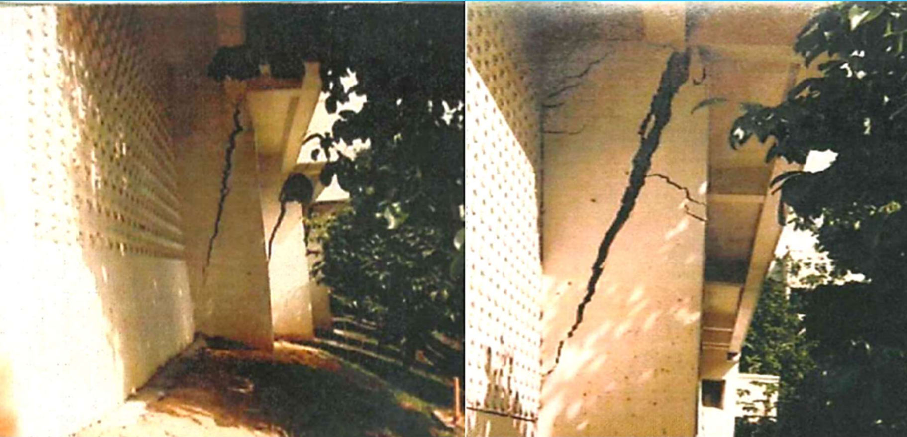
Views of carpark columns with large diagonal shear cracks
