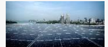
On-site PV + 100% REC off-set
