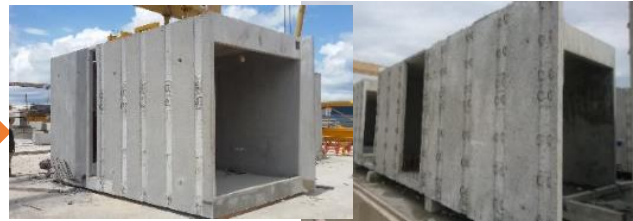
3D Module after casting
