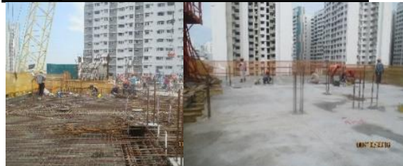
Preparation for Transfer Slab
