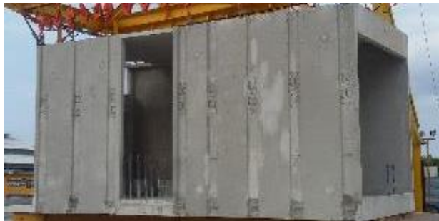
The Clement Canopy PPVC Carcass (box modular shape)
