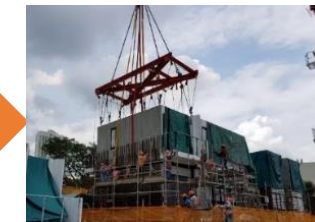
PPVC Module is installed
