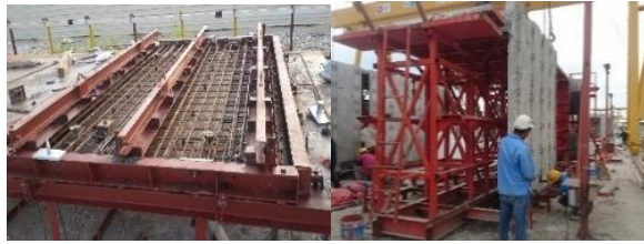
Panel fabrication / casting
