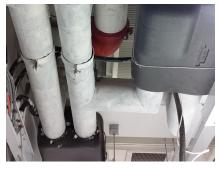
**Pre-insulated chilled water pipes** eliminate corrosion due to poor site quality control and save manpower by 30%.
