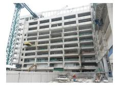
**Lightweight Precast Concrete Panels** (recycled content 30%) and prefabricated steel stiffeners. Improve productivity by 150%.
