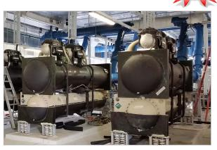
**Magnetic bearing centrifugal chillers** Rotating shaft levitating on a magnetic field eliminate mechanical friction loss and allow lubricant-free operation. Reduces maintenance costs and provides energy savings of up to 57%.
