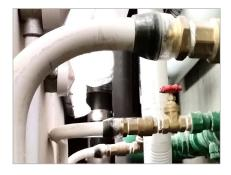
**"PEX" polyethylene water pipes** Light and flexible pipes that come in bundles are easy to handle and bend around obstacles and corners.
