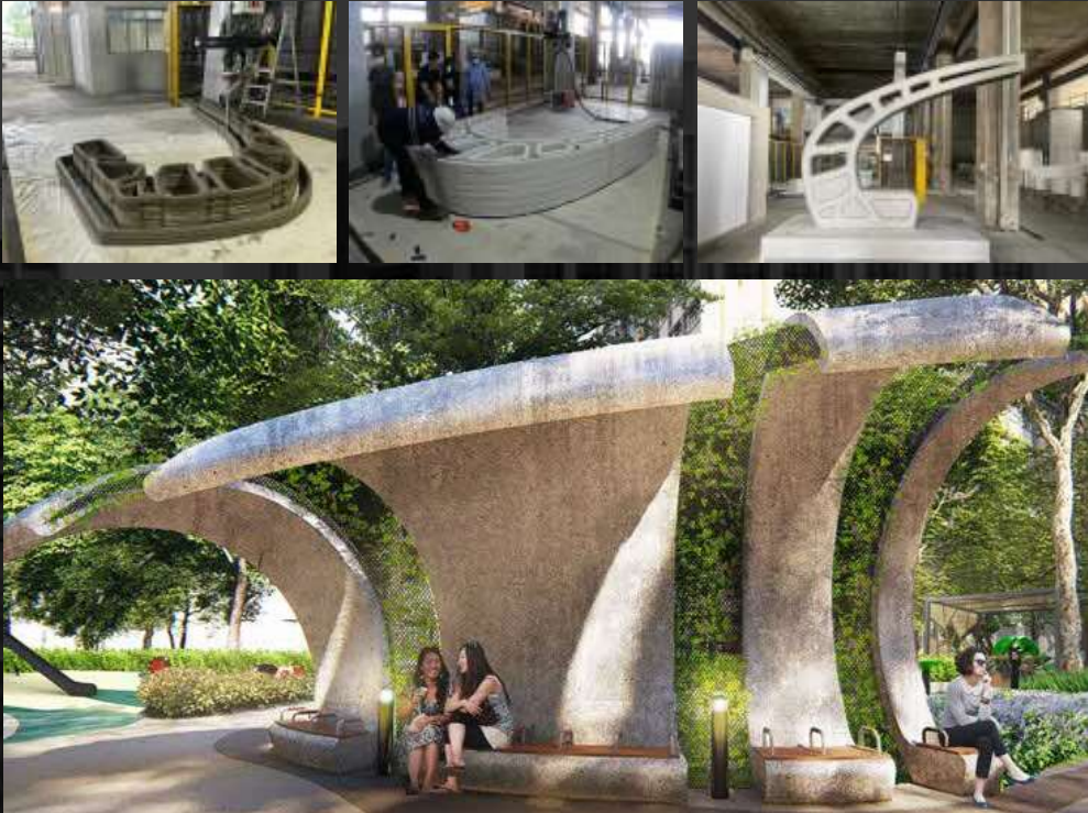
3D concrete printing to explore the creation & use of unique, organic-shaped benches Garden Waterfront @ Tengah
