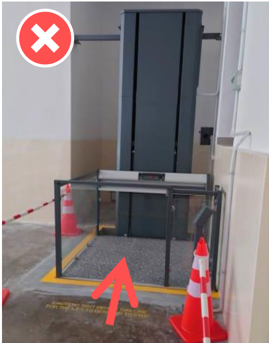
Platform lift without enclosure
