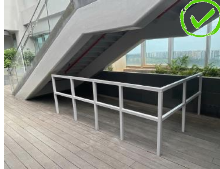
Addition of guard/barrier to prevent a person from walking near the space where headroom <2m.
