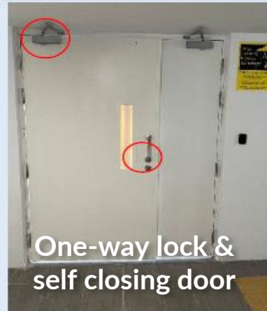
Figure H—VII: One-way lock and self closing door / gate; with a signage to indicate maintenance area
