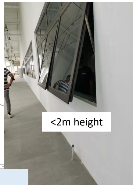
Addition of guard/barrier to prevent a person from walking near the space where headroom <2m.
