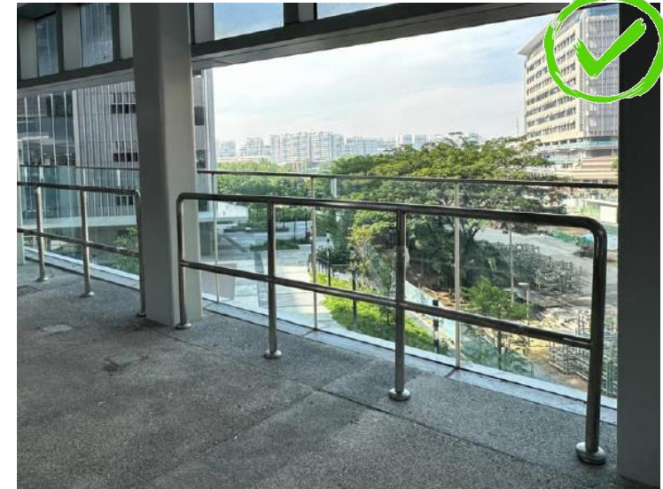
Addition of guard/barrier to prevent a person from walking near the space where headroom <2m.
