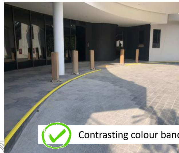
Tactile warning indicator with contrasting colour (no level difference)
