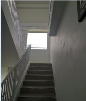
Figure H—V: Staircase to the Roof
