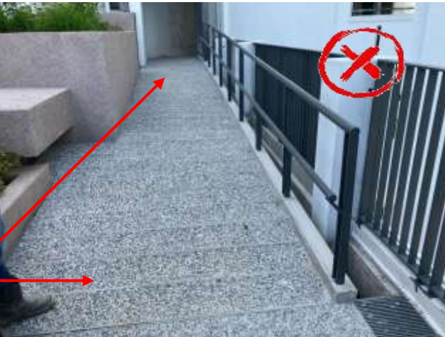
Gratings and gaps along accessible route >12mm
