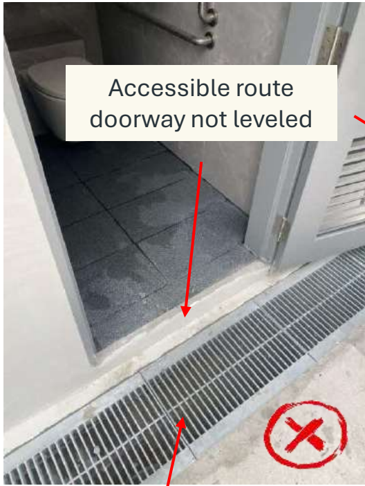
Gratings and gaps along accessible route >12mm
