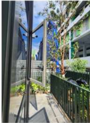
Window opens into circulation path <2.0m
