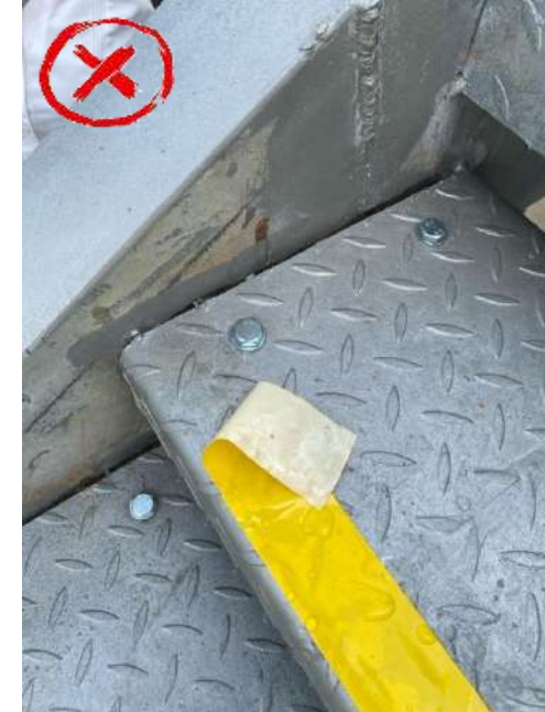
Tape is not an acceptable solution
