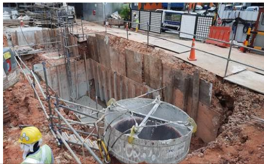
Inspection for any non-authorized works
