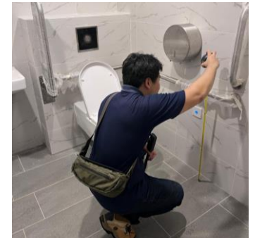
Checks on Accessibility Provisions
