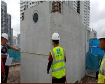
Checks that shelters are built as designed
