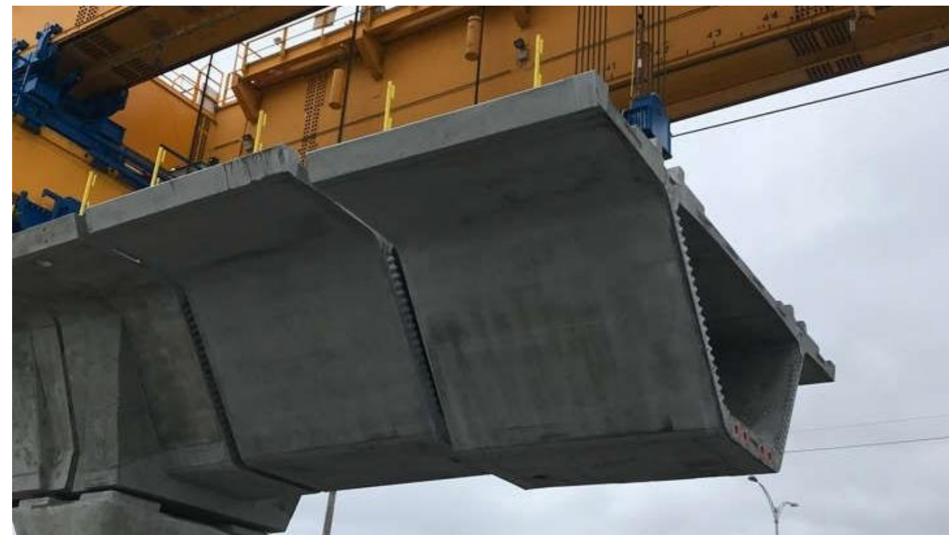
Inside box girders
