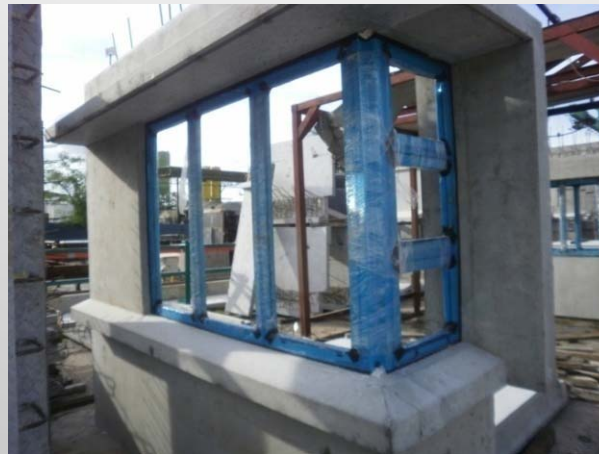
Completed precast unit
