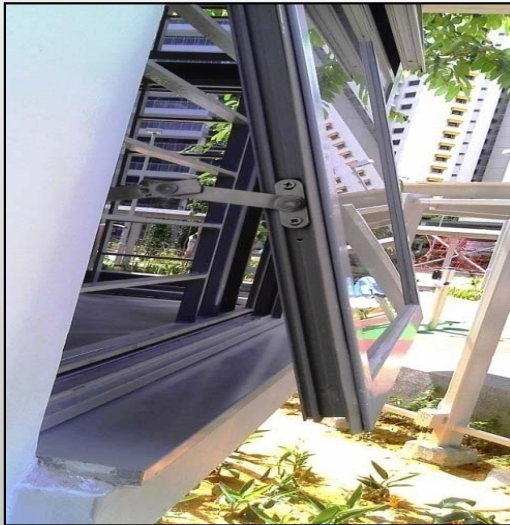
Stainless steel restrictor – restrict the opening angle.
