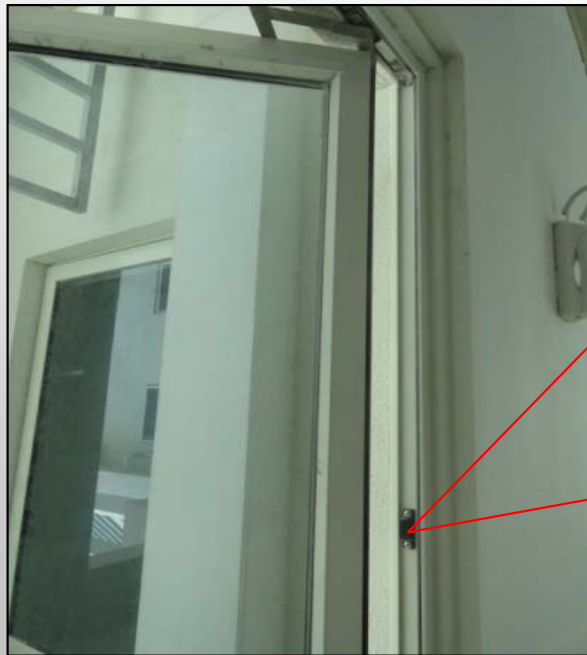
Part view of an casement window - installed with wind block.
