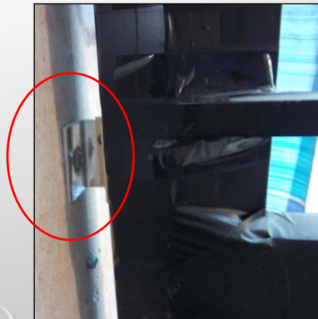
Fixing of primary bracket on wall
