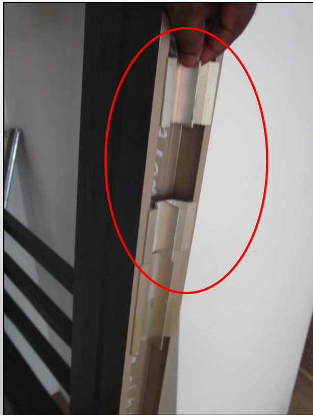
Extruded secondary bracket to outer frame
