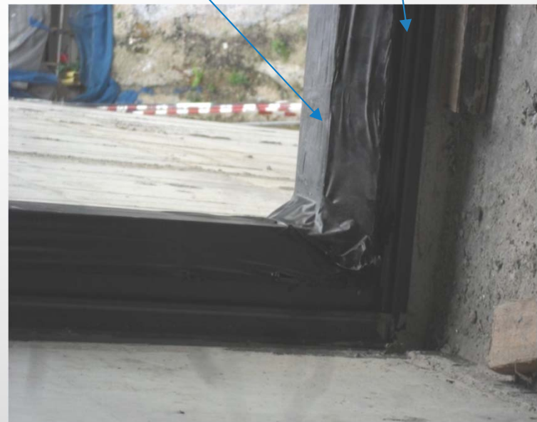
Install Inner Frame into sub frame
