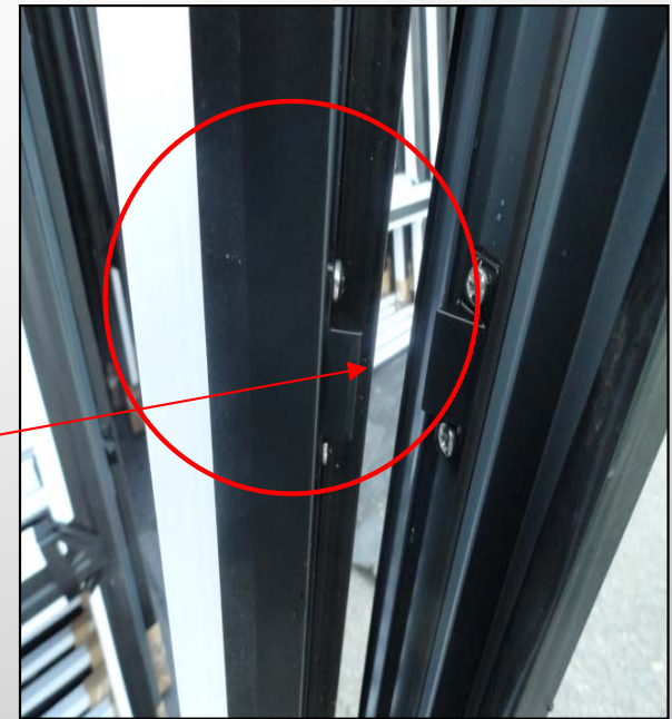
Wind block – resist buckling when subject to wind load.
