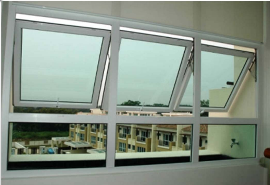
3 panels top hung window with fixed below.
