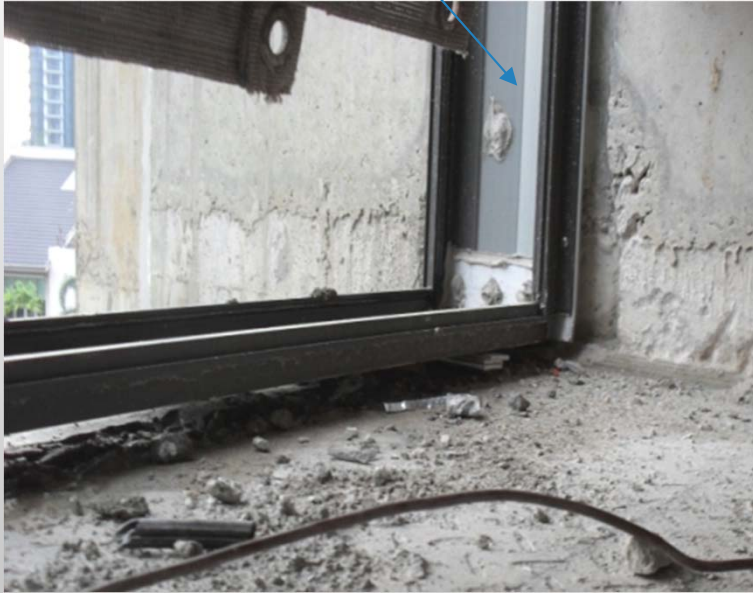
Installed Sub Frame - Window
