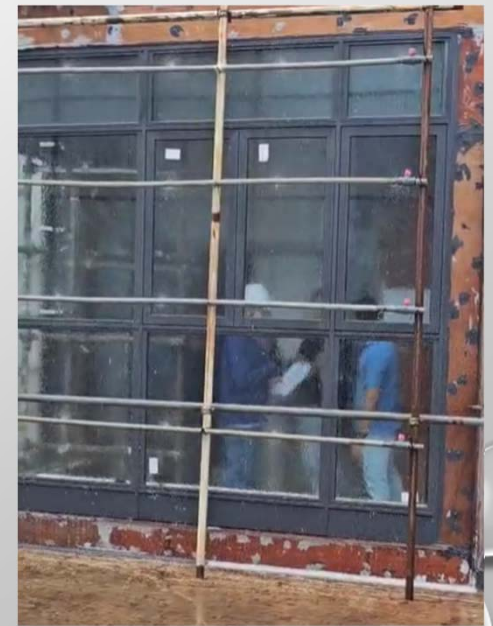
Water spray on façade.
