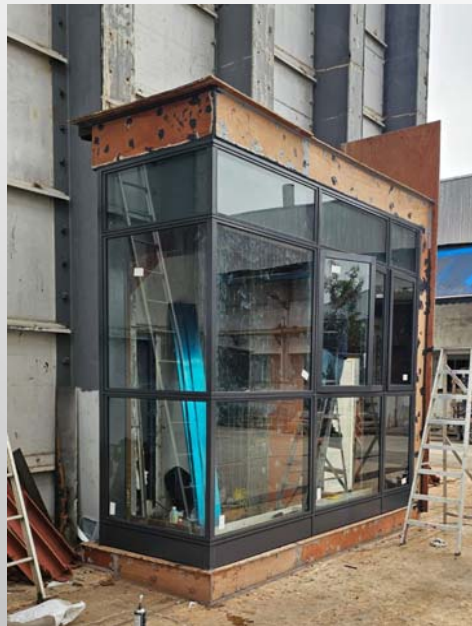
Window installed - Side
