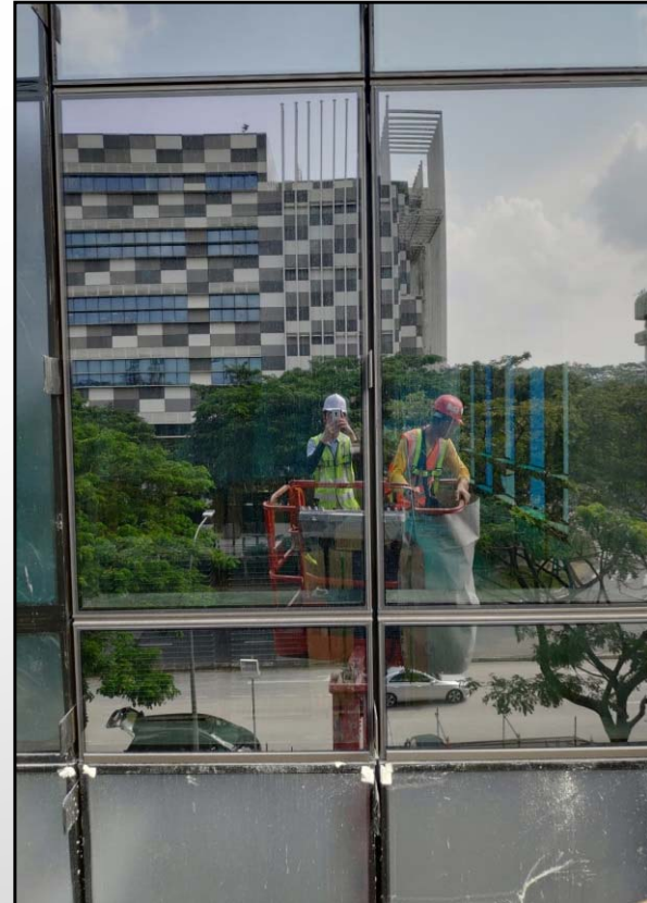
External view of the glass façade is acceptable.
