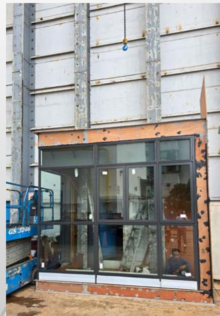
Window installed - Elevation
