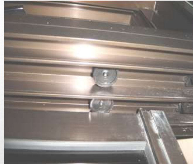
Safety device to prevent jumping track.
