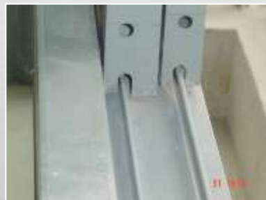
Bottom sliding track
