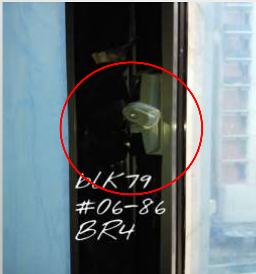
Broken Cam handle
