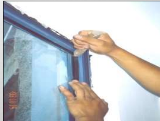
Gasket to be inserted and tool to tightness.
