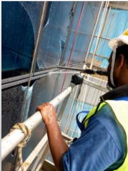
ASTM 501.2 Field water test – nozzle position at groove joint.
