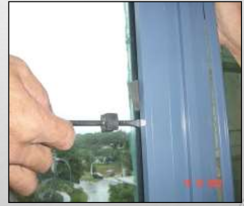
Insert block to secure glass
