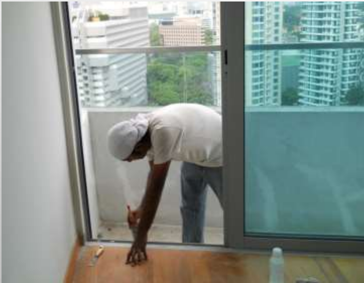
Cleaning of sliding bottom track.
