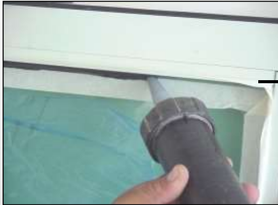
Application of silicone sealant to glass.
