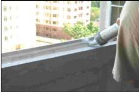
Install bottom frame and seal the gap
