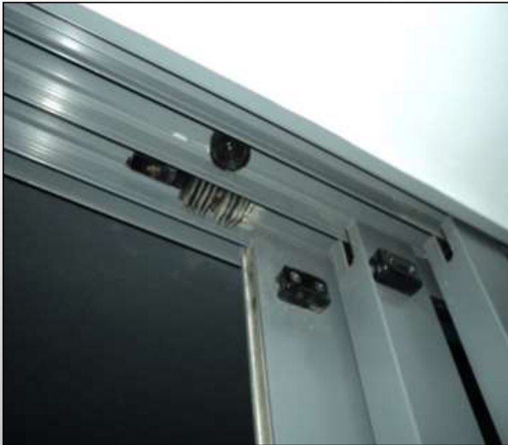
Window stopper to prevent jump track and Fall off.
