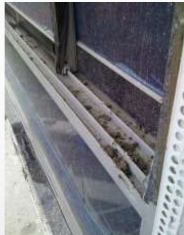
Sliding window bottom track stained with cement.
