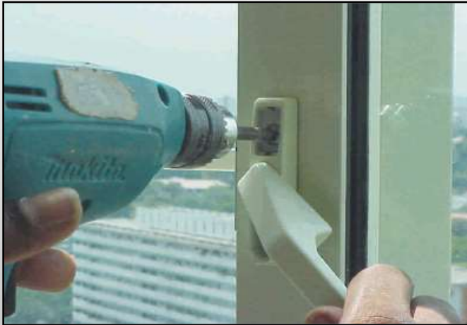
Installation of casement handle.
