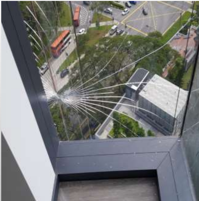
Point load on laminated / float glass.
