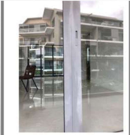
Colour fading on powder coating finishes.
