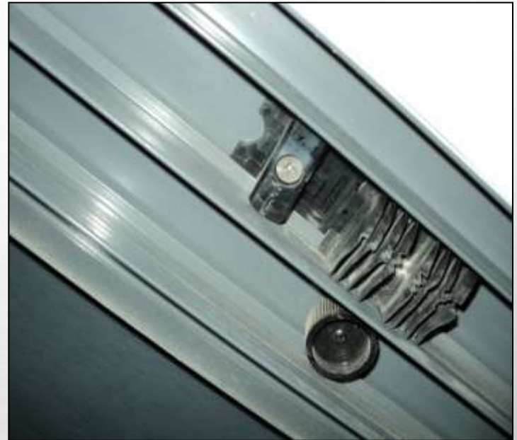
Wind block install on top track to reduce sound transmission, noise, particular windows that are facing MRT tracks and highway.
