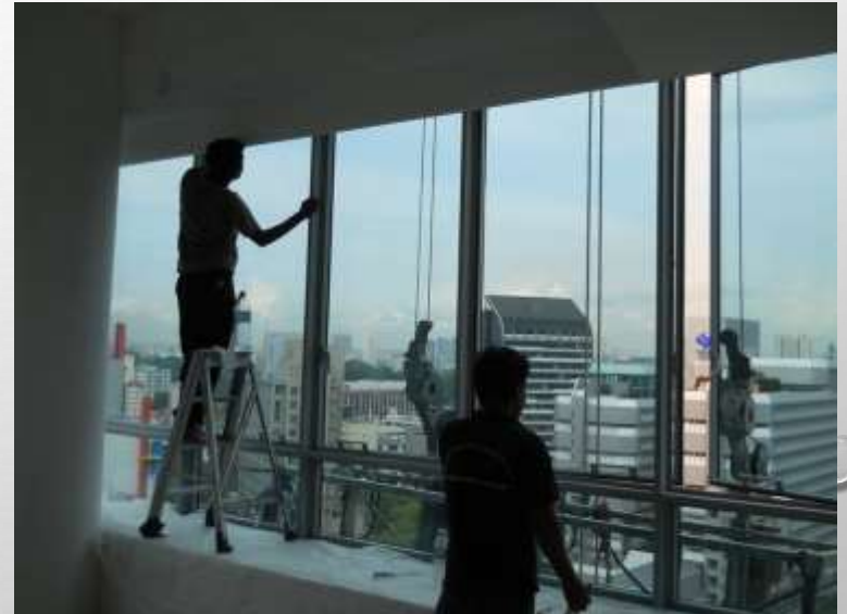
Cleaning of window, both external and internally .
