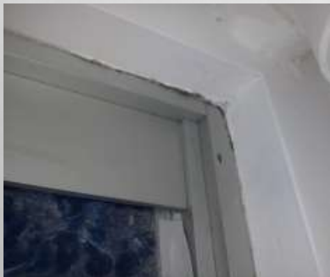
Before installation – dirt and debris must be cleaned.
