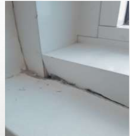
Dented bottom outer frame.
