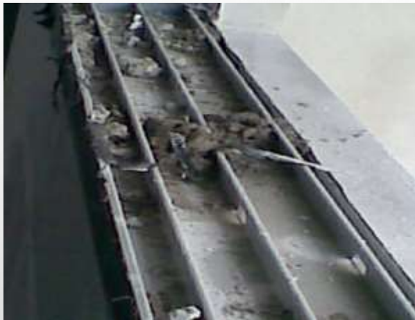
Before installation – dirt and debris must be cleaned.
