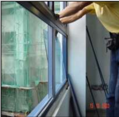
Inserting glass panel
