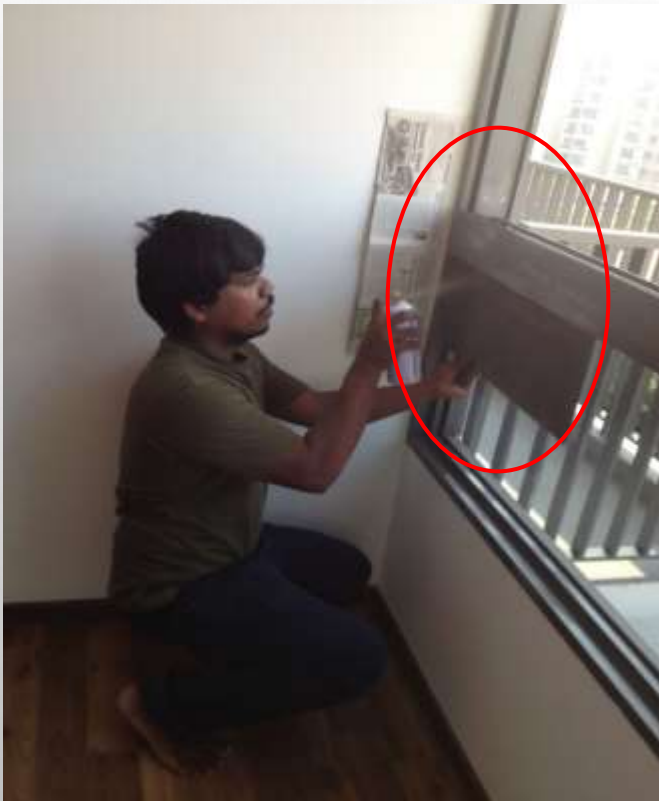
Touch up works – manual hand spray over powder coat surface.
