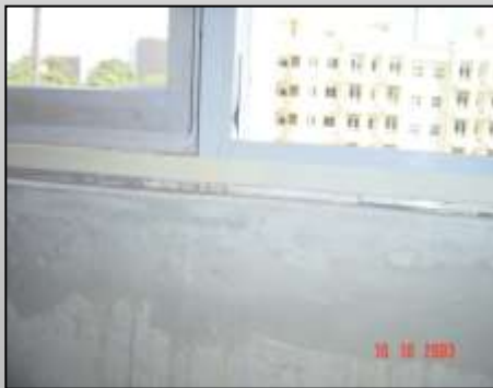
Protection with masking tape
