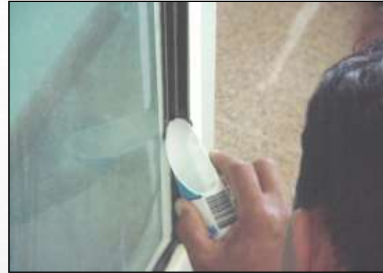
Use custom made tool to achieve consistent / desire surface finish.
