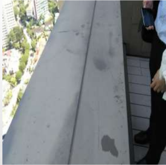
Colour fading on powder coating finishes.
