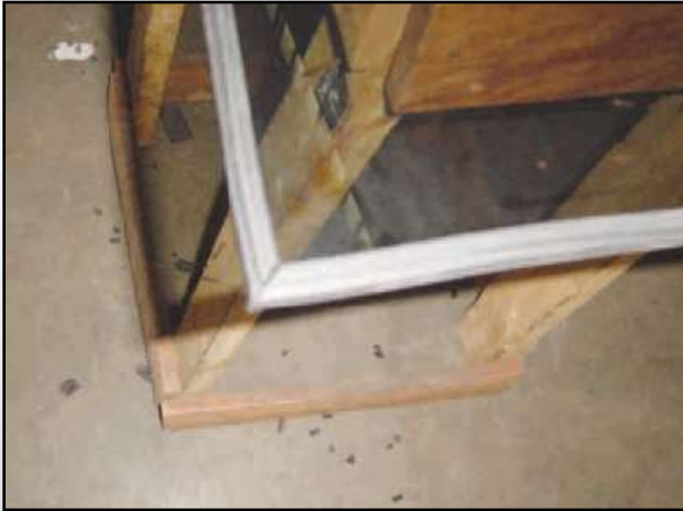
Step 1 – Insert gasket to glass.
