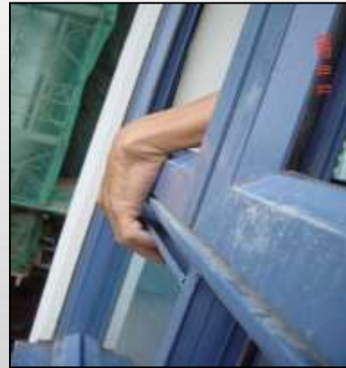
Secure of horizontal beading
