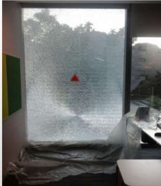
Shattered due to presence of impurities
