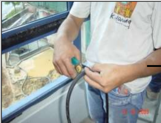
Preparation of gasket insert.
