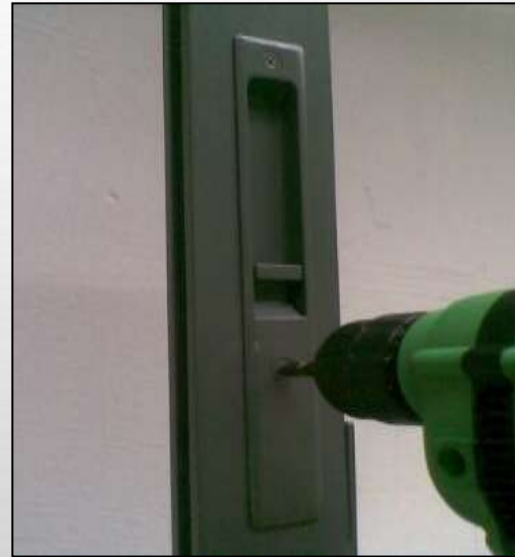
Installation of latch lock to window frame.
